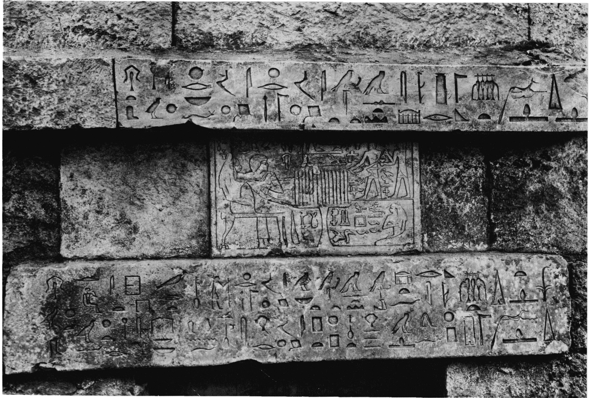
MASTABA OF KHWTA Lintel of the entrance.
