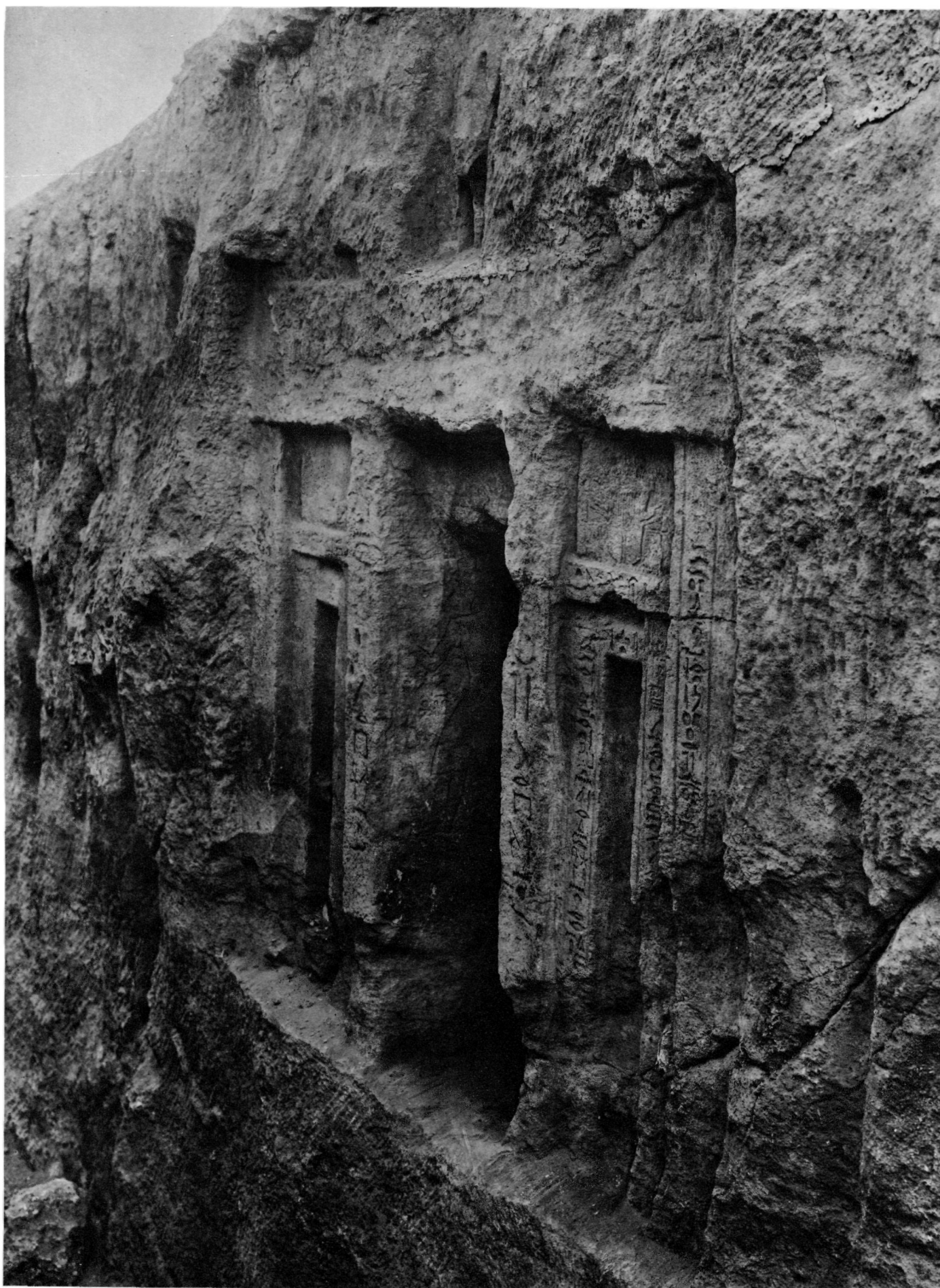
MASTABA OF MER-ANKH-F The façade.
